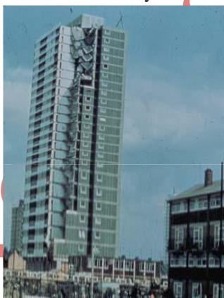
Fig.7: Progressive Collapse Ronan Point, UK, 1968[3]
