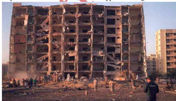
Fig. 4 a) Khobar Towers, US Marines HQ, Saudi Arabia, 1996 Explosive, 9 ton TNT equivalent, standoff, 25m 19 victims, 450 injured,
